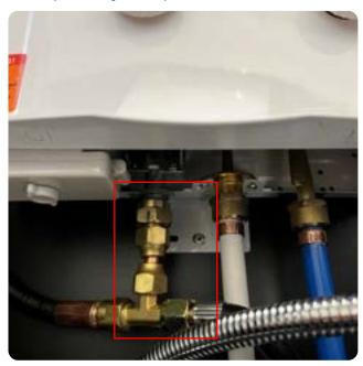
**Note:** Check regularly for leak, this can be done with soapy water. Due to the rugged use of the trailers in off road conditions. Vibrations can cause loosening of connections.
