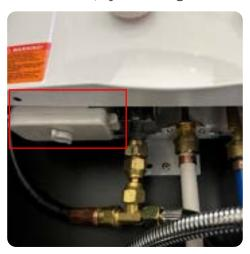
3. Drain the water heater and open the pressure relief valve to assist in draining. This is the brass tube located to the right of the middle of the unit. Leave this out over the winter.
