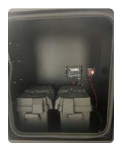
**Note:** Setting up the optional Renogy batteries requires a Bluetooth-enabled phone or tablet along with the Renogy app. One of the batteries must be designated as the master, and upon installation, the batteries are linked together, appearing as a single 200 Ah capacity cell when monitored through the app. For detailed instructions, refer to the manual provided by the manufacturer.
